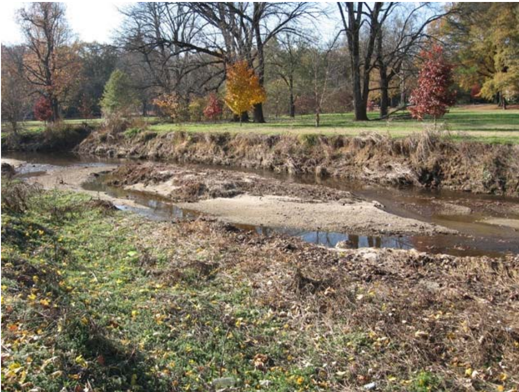
Figure 10: Enlargement of channel due to urban runoff, Lower Latham
