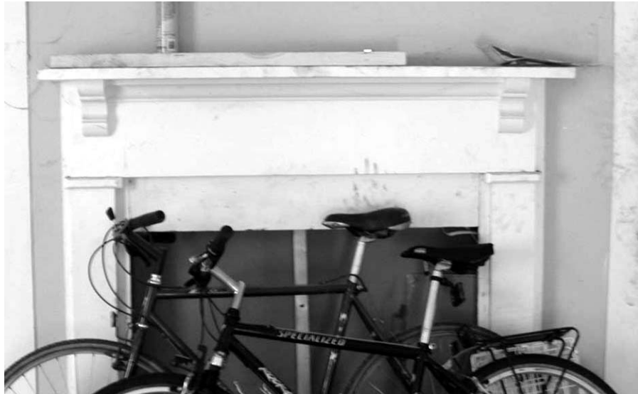
Figure 32: Original mantle located in House C; the firebox and chimney behind it were removed. Photograph by the author, 2003.
