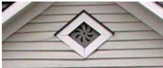
Figure 21: Decorative gable vent from the façade of House I, the only original architectural embellishment. Photograph by the author, 2005.
