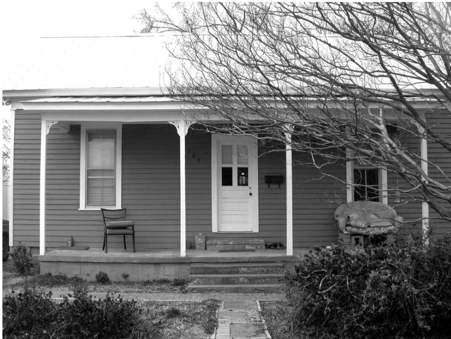
Figure 30: House B, with original style posts and Victorian scrollwork details. Porch floor has been replaced with concrete since 2002. Photograph by author, 2005.
