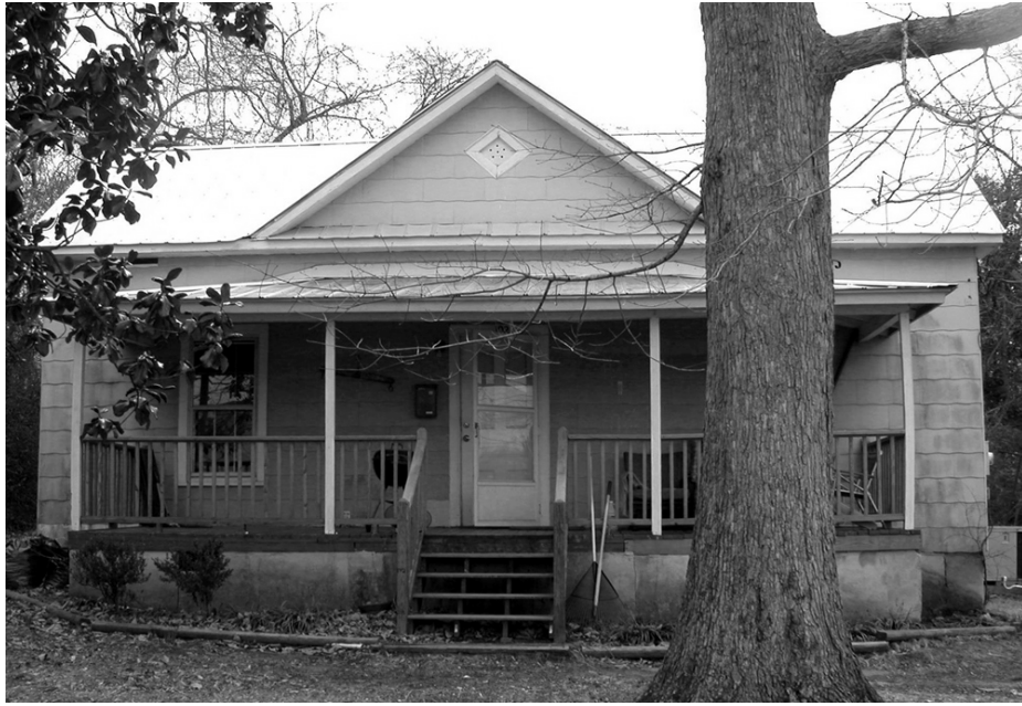
Figure 29: House E, with original style porch posts and newly added railing. Photograph by author, 2005.
