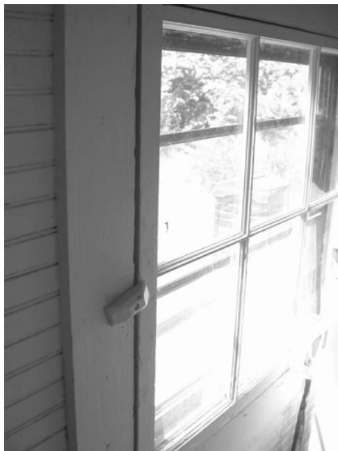
Figure 25: Window in enclosed back porch of House C. It is half of a double-hung window used as a casement; note wooden latch closure. Photograph by author, 2003.
