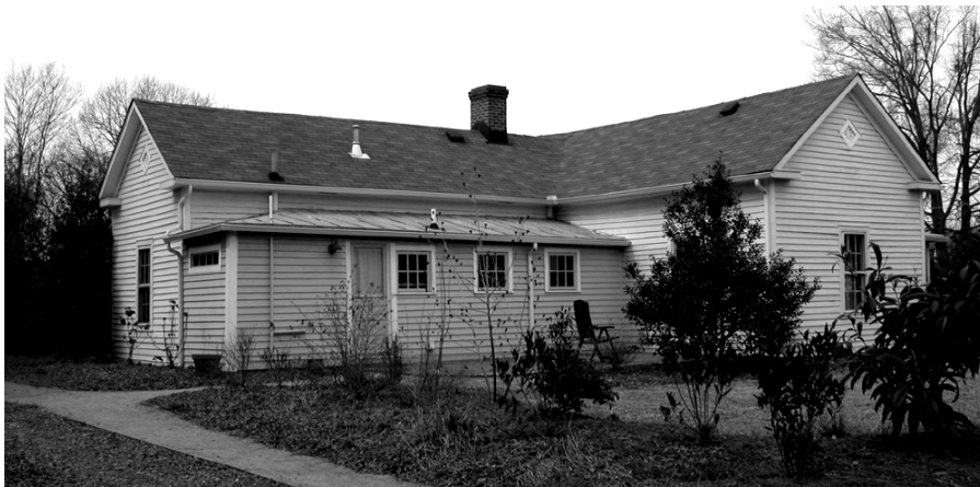
Figure 23: Rear side of House F showing the enclosed back porch. Photograph by author, 2005.
