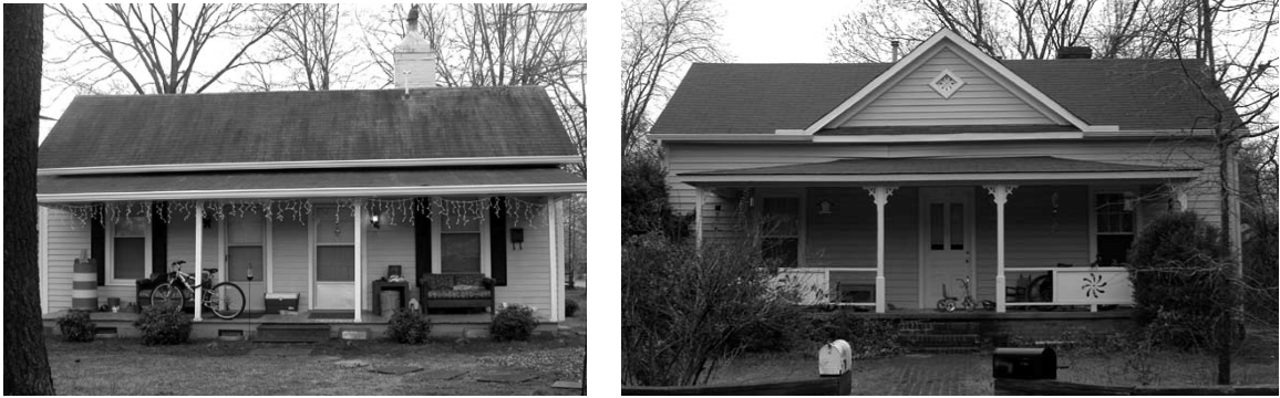
Figure 16: Examples of the two house types apparent in Carrboro. On the left, the saddlebag house with two front doors, on the right, the three-gable house with a single door.
