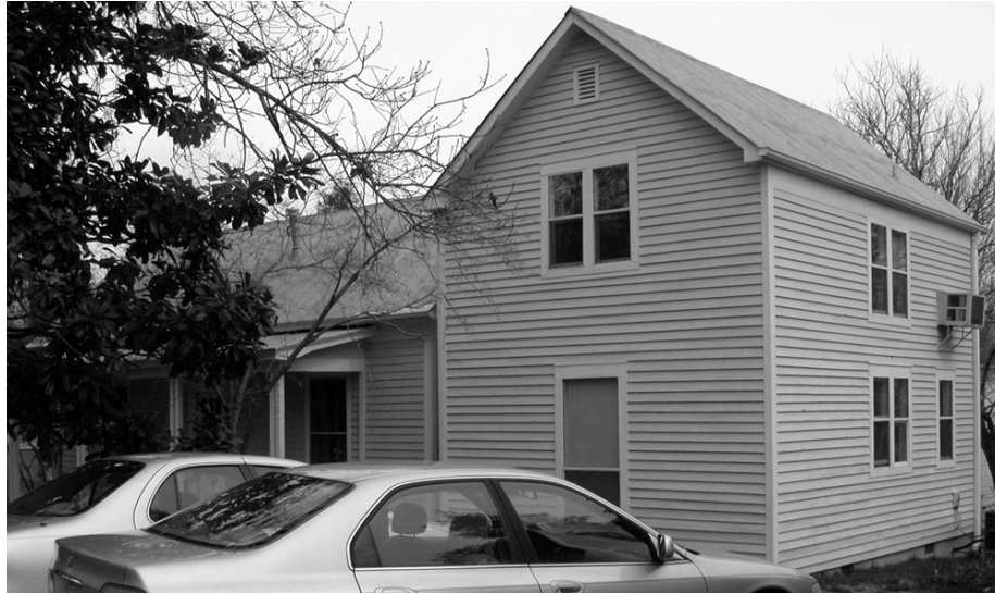
Figure 28: Two-story addition to south side of House J, the only mill house altered with a side addition and a second story. Photograph by author, 2005.
