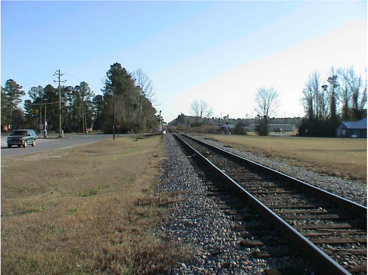
Figure 28. This photograph shows a view looking south at Rose Hill towards the bluff of the scarp on the route of the Wilmington & Raleigh Rail Road. The rails follow the topography without extensive excavations or embankments. Photograph by James C. Burke
