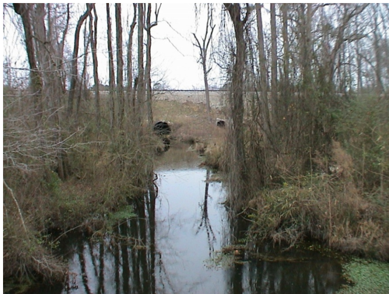
Figure 6. The most extensive embankment on the Wilmington to Faison section of the Wilmington & Raleigh Rail Road is at Bear Swamp, a short distance from Faison. It was originally trestlework, and was filled in during the renewal of the road in the 1850s. Photograph by James C. Burke
