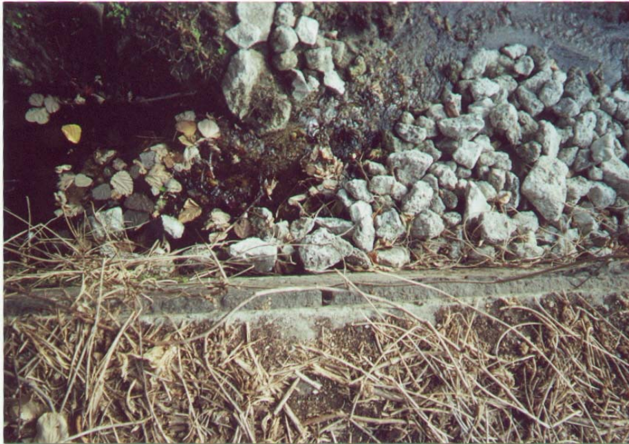
Figure D1. The stream running through the ravine of the railroad cut at Wilmington is still visible east of Fourth Street. Photograph by James C. Burke
