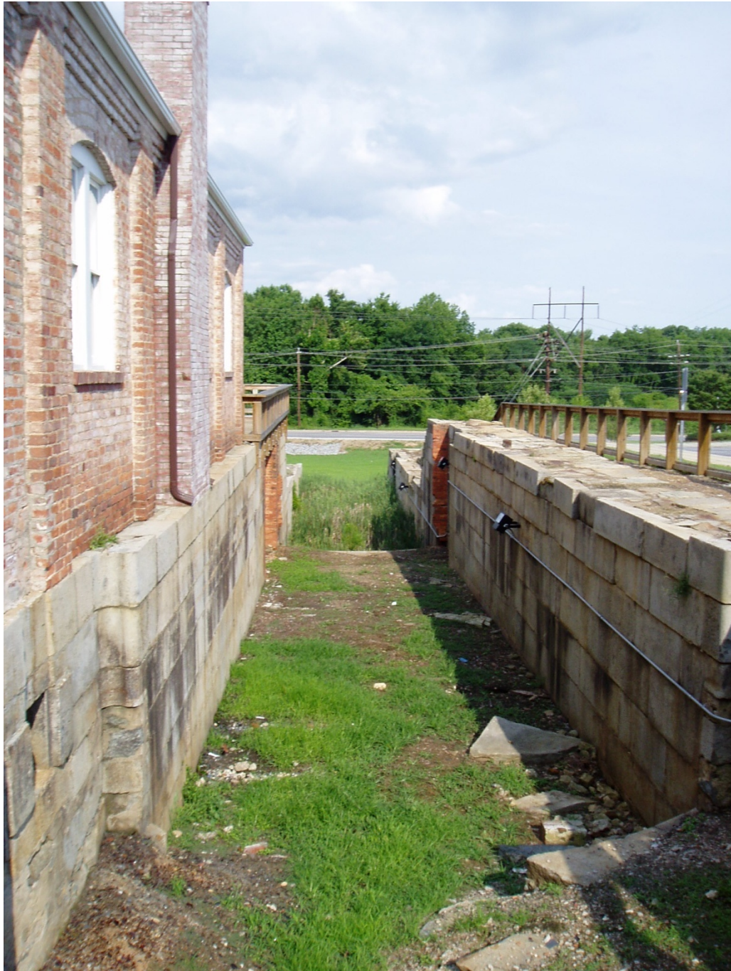
Figure 11. The remains of the upper locks of the Roanoke Canal are located at Roanoke Canal Museum in Roanoke Rapids, North Carolina. The narrow width of the locks was designed for bateau, a shallow-draft boat of about eight feet in beam. The bateau could carry ten to twelve hogsheads. Photograph by James C. Burke
