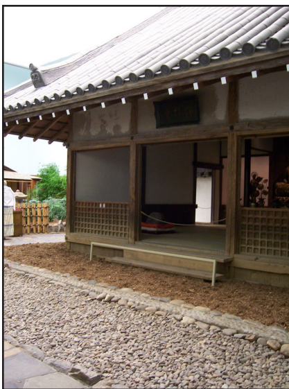
Figure 3.25: Temple of attainment, few physical barriers keep visitors out
