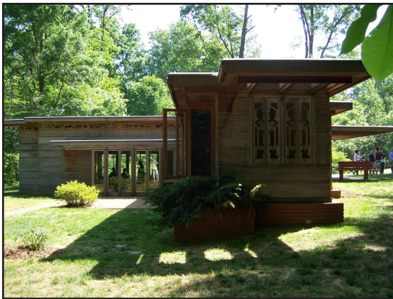
Figure 3.11: East exterior view of Pope-Leighey house
