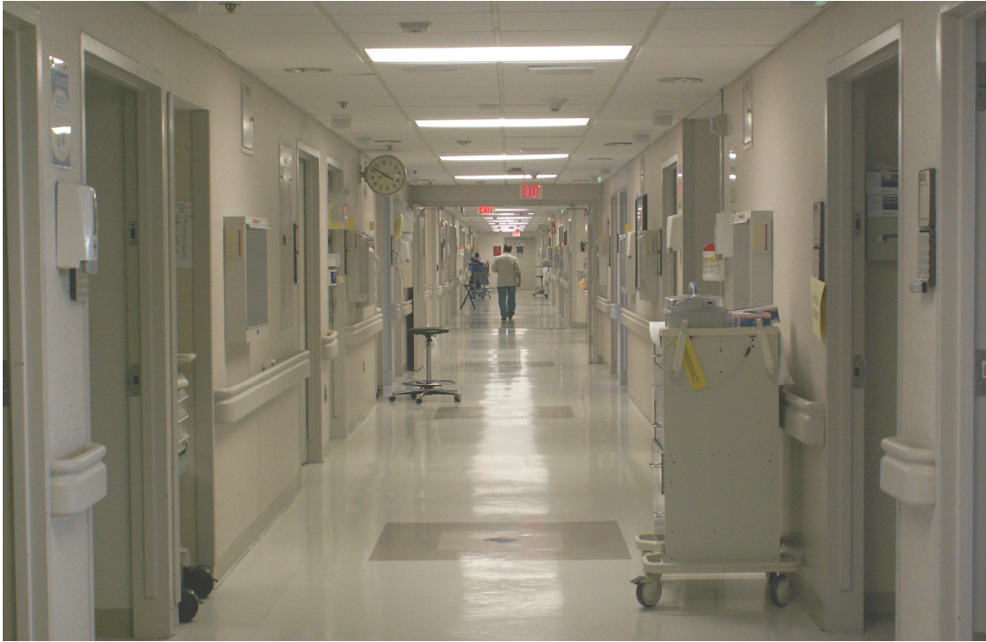
Figure 7. Existing 5 th floor corridor, typical.
