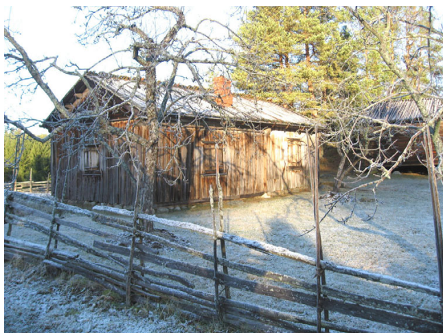
Figure 10 The croft of Paikkari, Sammatti, in the south of Finland, was a typical building in the countryside. It was built in 1799–1800 and enlarged by a later owner in 1825. In the more developed parts of Finland chimneys were common, but in the poorer parts of the country the smoke was led out from the building by a hatch in the roof. Originally the croft was a one room (ca 6 × 6 m) log cabin and the birth place of Elias Lönnrot (1802–1884), who collected the Finnish national epos Kalevala. The household consisted of nine persons. The separate sheds were not warmed. Lönnrot's father was a parish-tailor. The family belonged to the stratum under the farmers, but socially represented the crofters, that were the highest group of the non-landowners. The picture is taken in November (2007), the soil is already frozen and the sun is above the horizon for 5 h and 30 min.
