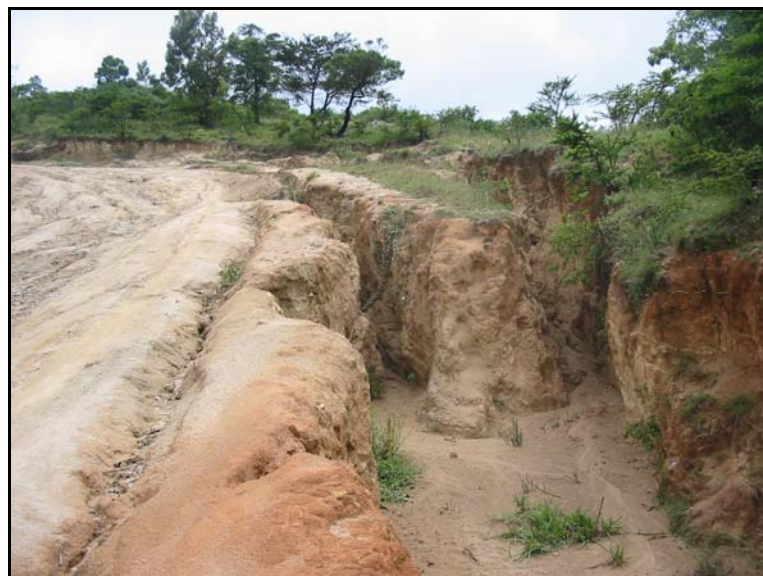
Figure 16. Gully erosion site along the road (Keskinen 2005).
