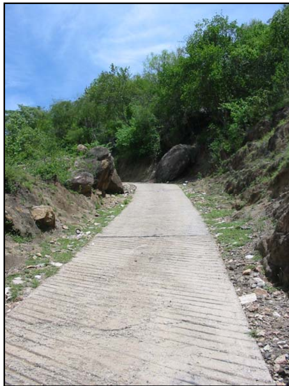
Figure 18. A steep road section paved with concrete surface (Keskinen 2004).
