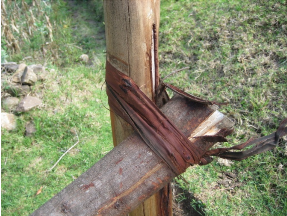
Figure 28. “Construction without nails” by using tree bark ( Acacia sp. ) (photo by Himberg 2009)
