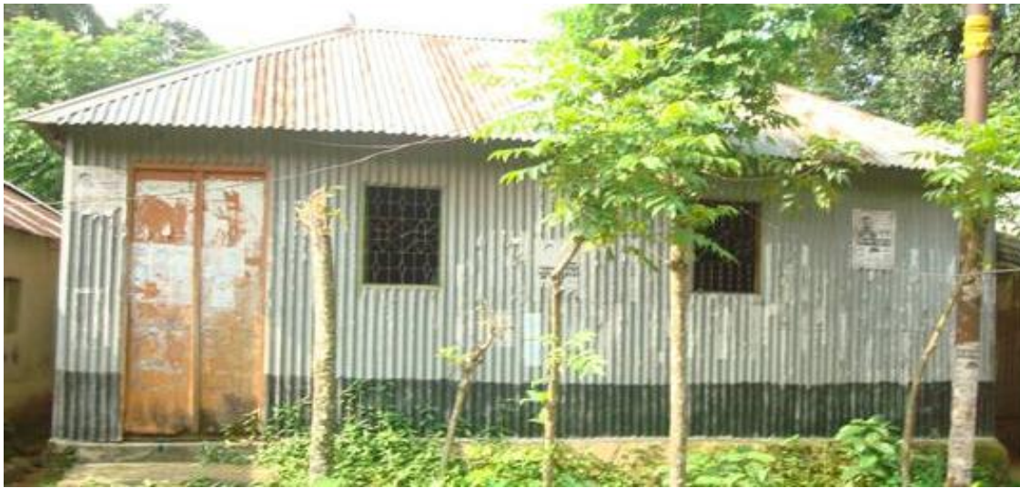
Fig. 10 A rural house; both the walls and roof are made of CIS
