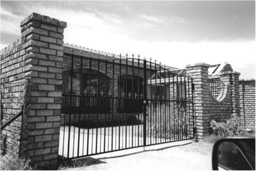
Picture 2: A thoroughly renovated Group A house
