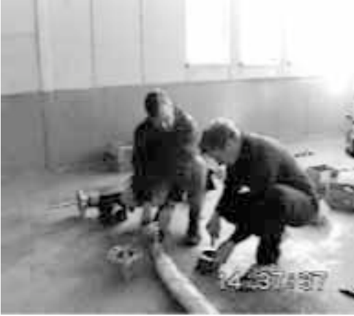
Figure 7.5 Assembling the flange joint for the oil-removing machinery
