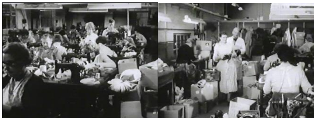
Figure 2-5. Original Closing Room. 166
