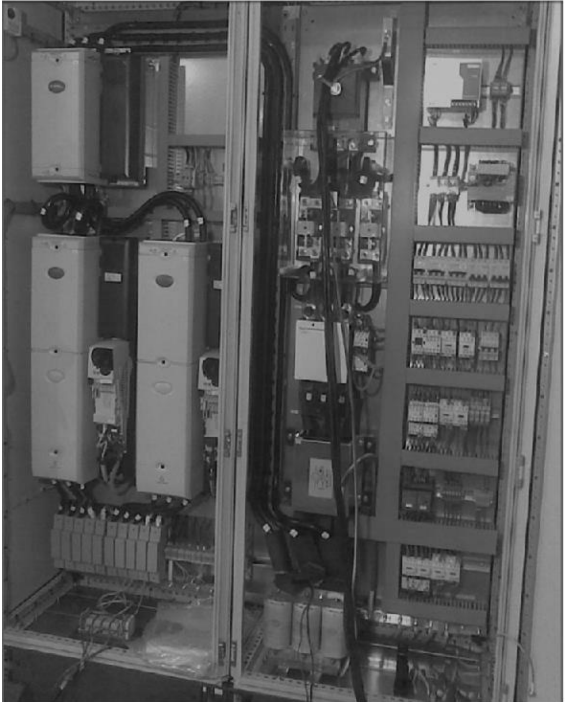
AC Drive & Control Cubicle Suite Photo ( Typical )
