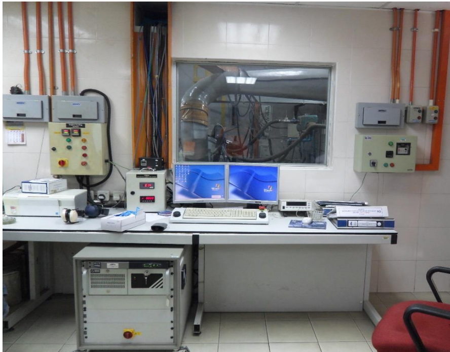
Fig. C Engine-dyno control room.
