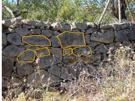
Fig. 5. Wall in the Algarvian barrocal , where one sees the technique “one on two” (Source: authors)
