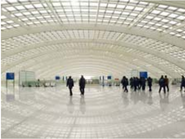
Fig.XVII Beijing Capital International Airport (Foster Associates 2004-08)
