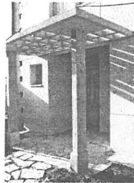
Picture1. South facade and atrium
