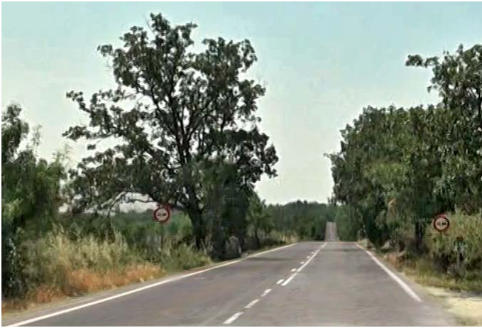
Figure 5. Real view of hidden dip on straight alignment
