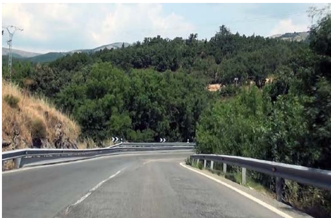
Figure 3. Real view of curve where sight distance is limited by vegetation.
