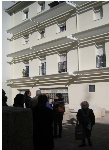
Fig. 4 South facade after renovation. December morning
