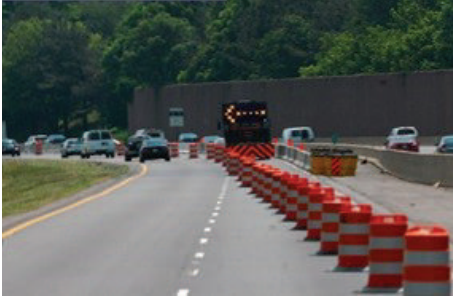
FIGURE 1: Example of a work zone delimited by barrels.
