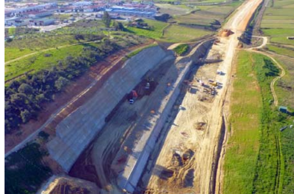
Figure 10.- View of upper and lower anchored walls
