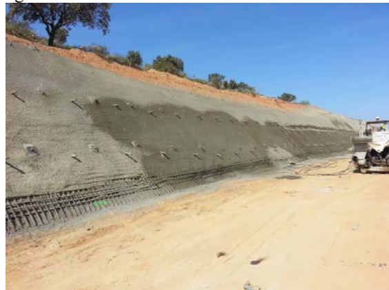
Figure 7.- Anchored wall wader execution
