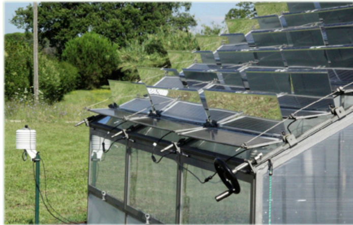
Figure 3. Greenhouse with mobile panels [65].
