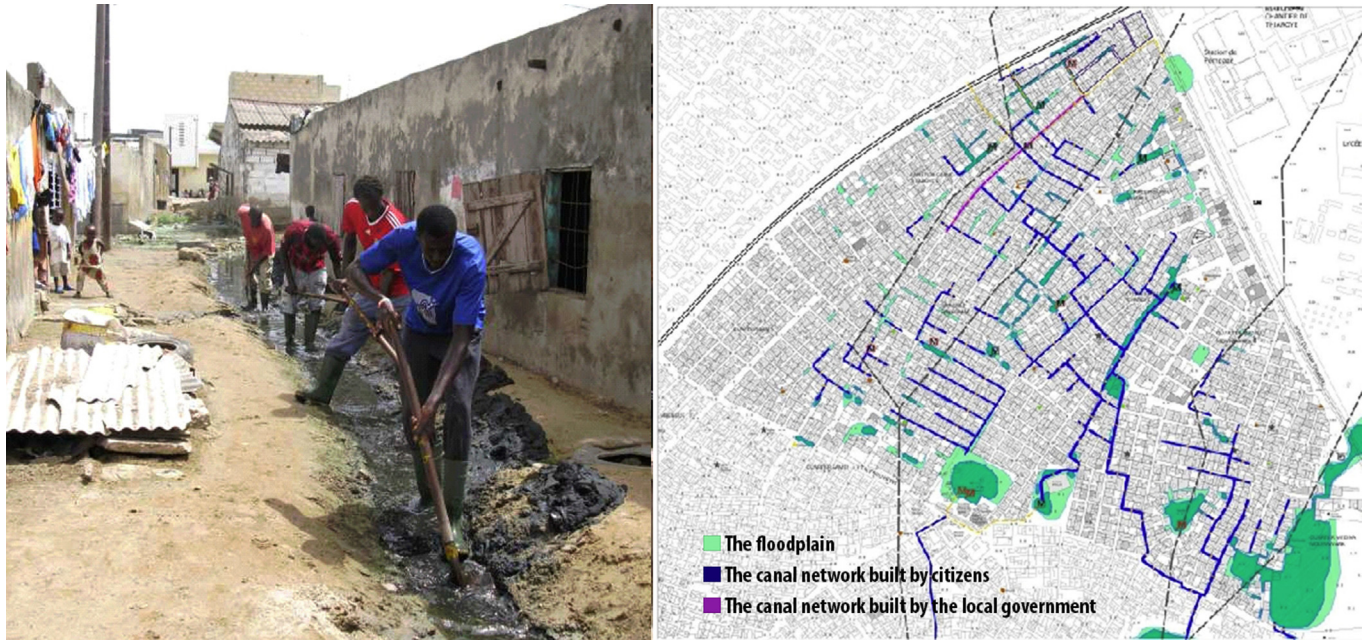
Fig. 4. Drainage system built by citizens. Source: Authors.
