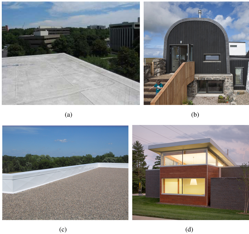
Figure 14. Examples of the different roof edges tested. (a) Simple edge; (b) curved edge; (c) railing; (d) cantilever.
