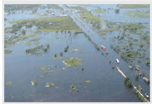
Fig.1: Federal road 180D totally submerged. Transit problems complicated evacuation and emergency aid activities. Source: CENAPRED
