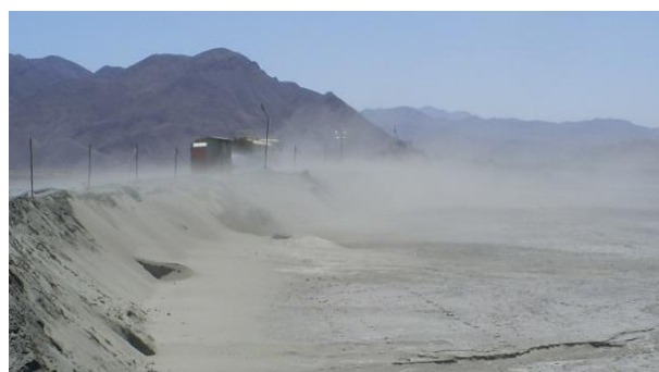
Figure 2. Erosive effect of wind on a tailings dam. Source: Self-elaboration, 2006.
