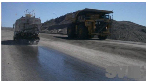
Figure 6. Applying particulate matter abatement product on unpaved roads. Source: Vial Corp S.A., 2012.
