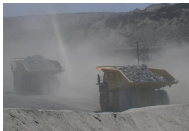
Figure 3. Particulate matter emissions from unpaved roads. Source: Vial Corp S.A., 2012.
