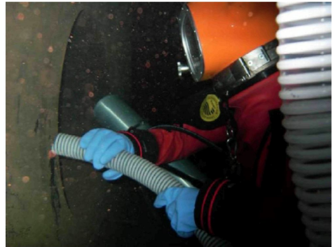
Fig. 4. Suppression pool cleaning.
