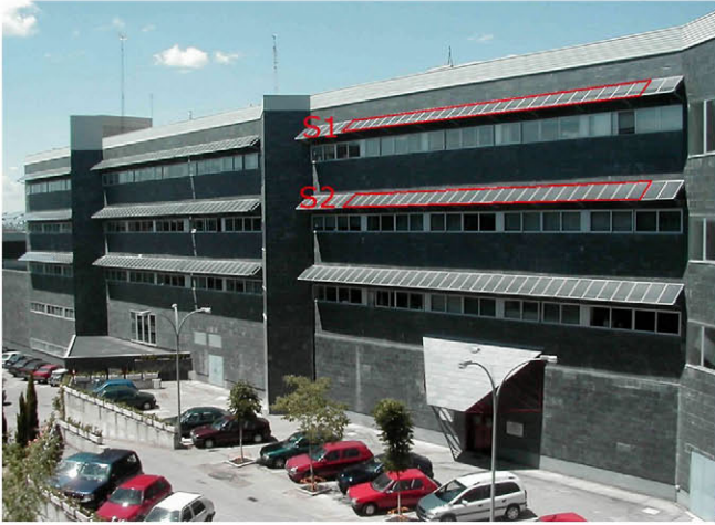
Fig. 3. PV system located on “Edificio López Araujo” building at ETSI. Telecomunicacion Madrid. (For interpretation of the references to colour in this figure caption, the reader is referred to the web version of this paper.)
