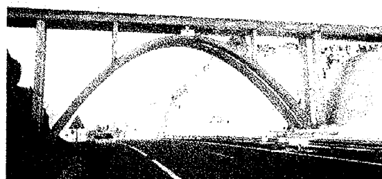
Figure 8. Arch Bridge in Solares, Santander
