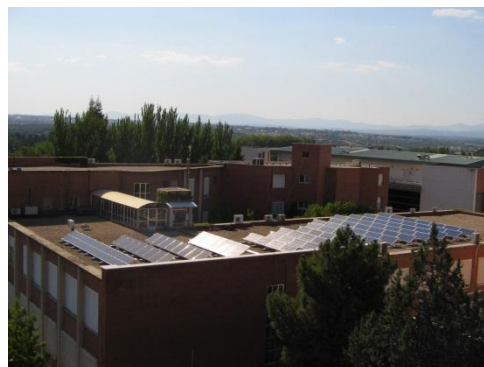
Figure 1: Roof of the building where the solar plant is located.
