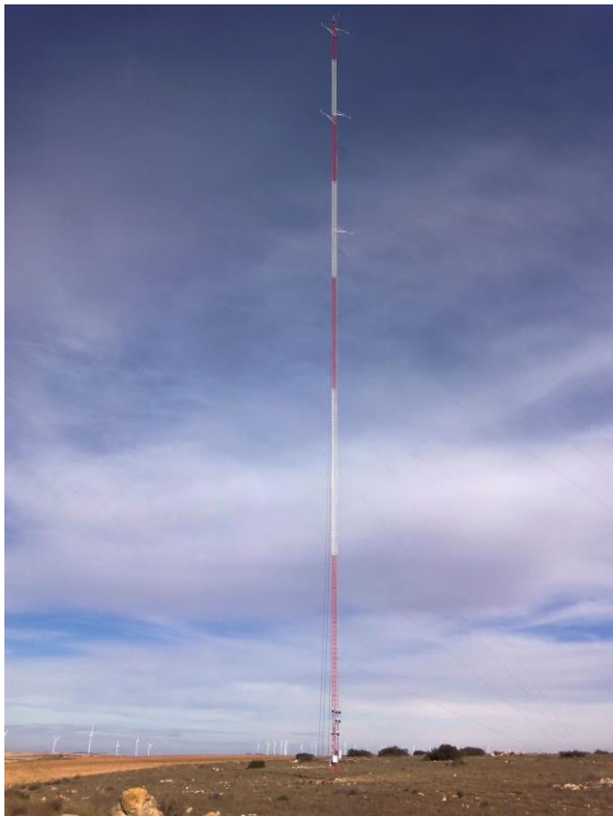
Fig. 6. Kintech Engineering meteorological tower located at Zaragoza (Spain).
