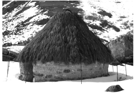
Figure 2. Braña in Asturias. Stone walls with straw roof in which the relation among the building material, economy and architecture is clear (María del Mar Barbero Barrera).
