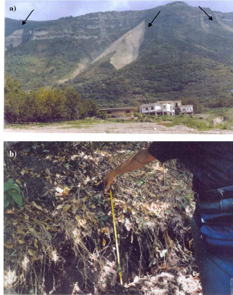
Figure 1. Examples of landslides occurred at Pizzo d'Alvano massif on May 1998: a) slides evolved into a landslide of the flow type; b) in the same are, an example of slide not evolved into a flow.
