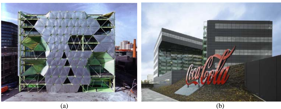
Fig. 4 (a) Media-TIC offices building. Barcelona (Spain), 2010, Cloud 9; (b) Coca-Cola Headquarters, Madrid (Spain), 2009, De Lapuerta and Asensio, The building has achieved a gold LEED certificate.
