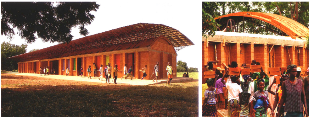
Fig. 6 Primary school extension, Gando (Burkina Faso), 2008, Diébédo Francis Kéré.
