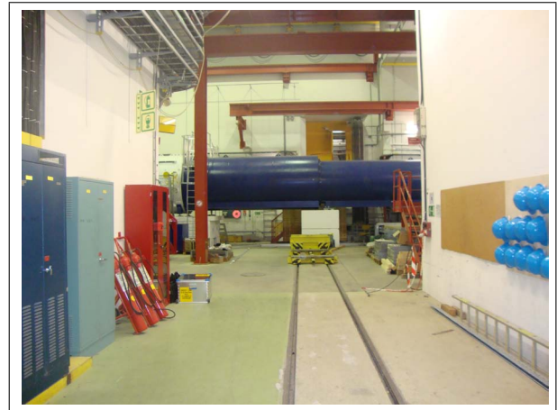
Figure 3. ECN3 tunnel area at CERN - view from the tunnel entrance
