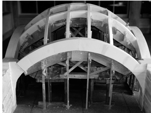
Fig.8: The crossing vault all ready built with the centering.
