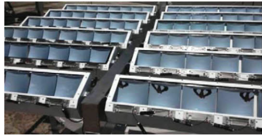
FIGURE 7. Field demonstration 2.3-kW array mounted on a carousel-type tracking system.
