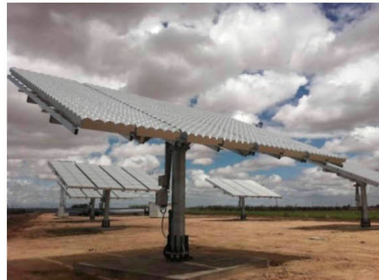
Fig. 6: CPV plant installed by BSQ with Daido modules in Villa de Don Fadrique (Toledo, Spain). Picture courtesy of BSQ.
