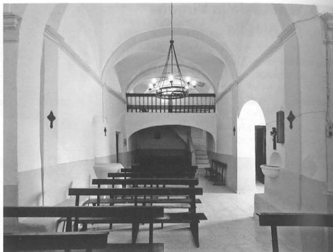
Vista interior nave.
