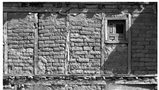
Figure 9. Timber reinforced wall in Zayas de Bascones. (Credits: Gil Crespo).
