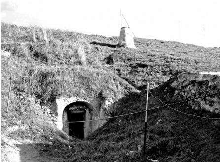
Figure 7. Outside image of a cave-dwelling in Valdaracete. It is dug on the slope and kitchen chimney can be observed as representative element as well as bioclimatic strategy. Source: Ignacio Javier Gil Crespo.
