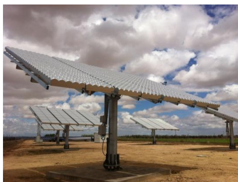
Fig 4. Overview of the 5 arrays installed in Villa Don Fadrique, Toledo (50kW installed). © BSQ Solar.
