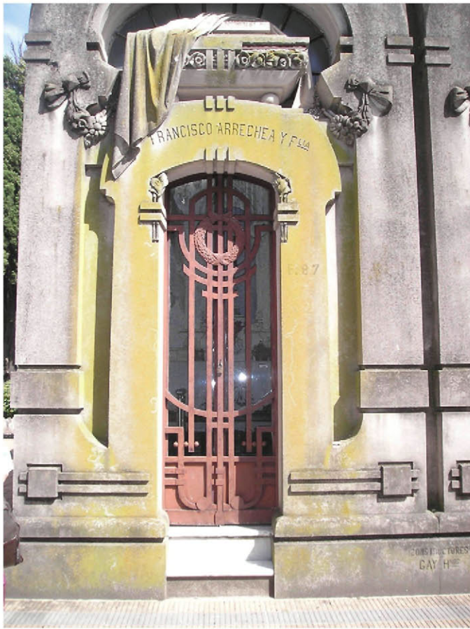
Fig. 1. Portico of the crypt of Francisco Arrechea (crypt F87), which is of architectural interest because of its Art Nouveau style. The yellowish coloration is indicative of the presence of Caloplaca austroctrina .
