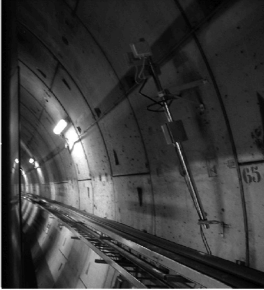
Fig. 1 Photo of a realistic circular tunnel in Madrid, Spain
