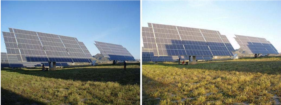
Figure 6. Shading profiles cast over 25 kW PV arrays of a commercial PV plant installed in Almería (Spain).
