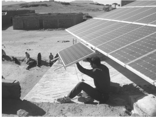
Figure 7. Reference module used as irradiance and cell temperature sensor.
