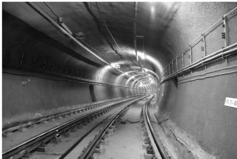
Fig. 3. Slab track installation
