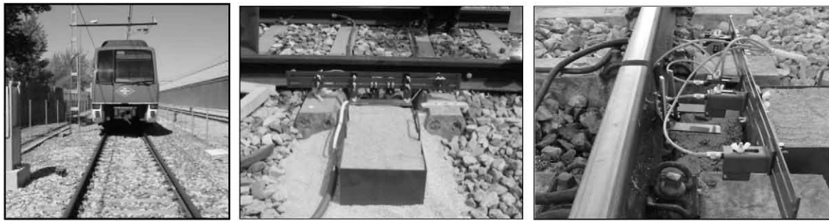
Fig. 14. The measuring equipment installed on the field testing site
