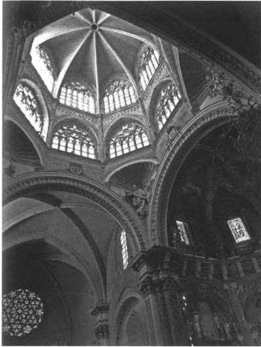
Fig. 3: View of the crossing from floor level.
