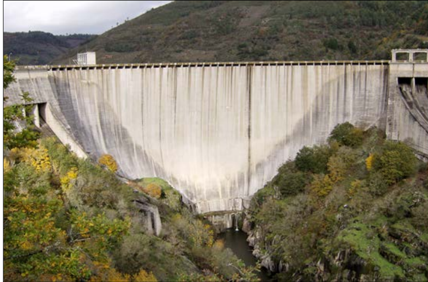
Figure 11: General view of the double curvature arch dam
