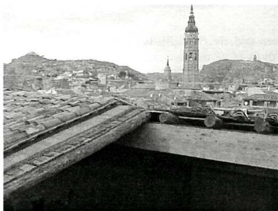
Fig. 3 – Roof restoration of the church of San Pedro de los Francos.
